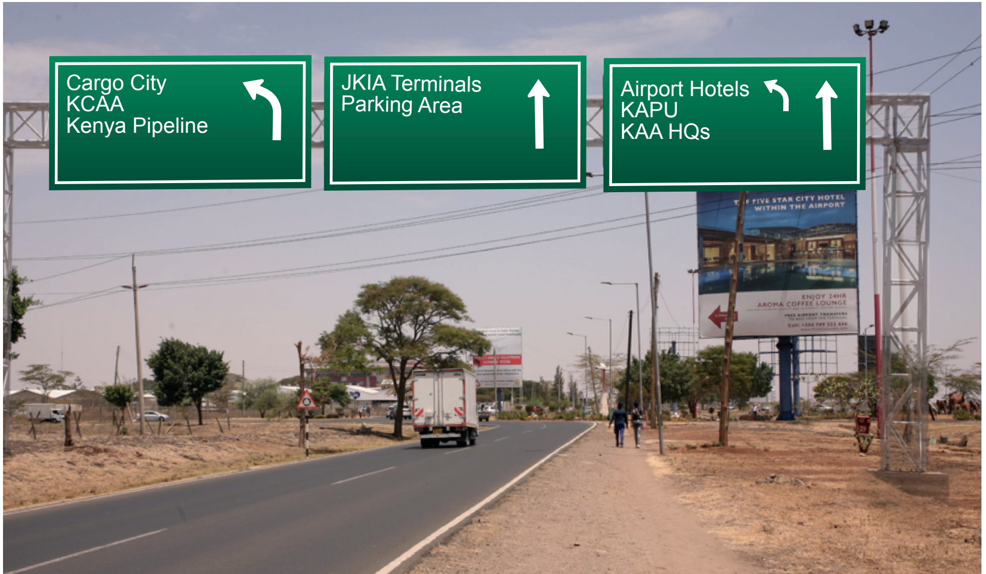
Gantries highlighting directions right from Mombasa Road clearly guiding people to the airport. The Signage and gantry is according to KENHA standards.
